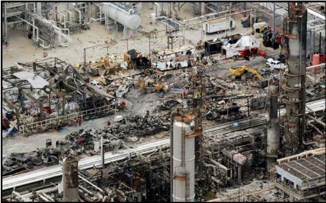
Figure 1. Refinery Explosion and Fire [6]
